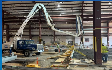
Existing concrete flooring removed and new reinforced concrete placements underway
